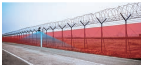
Airports Perimeter Security
